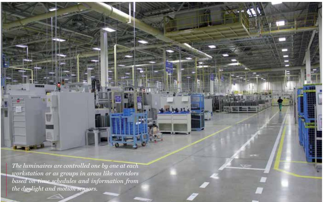
one at each workstation or as groups in areas like corridors based on time schedules and information from the daylight and motion sensors. For example, at lunch hour the corridors are lit brighter and the workstations are dimmed down. The system can be programmed in daily, weekly and monthly basis up to 5 years in advance, with planned downtime and holidays.
