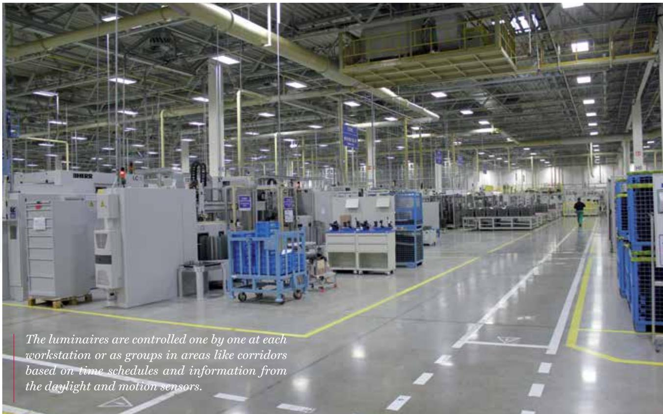
*The luminaires are controlled one by one at each workstation or as groups in areas like corridors based on time schedules and information from the daylight and motion sensors.*
